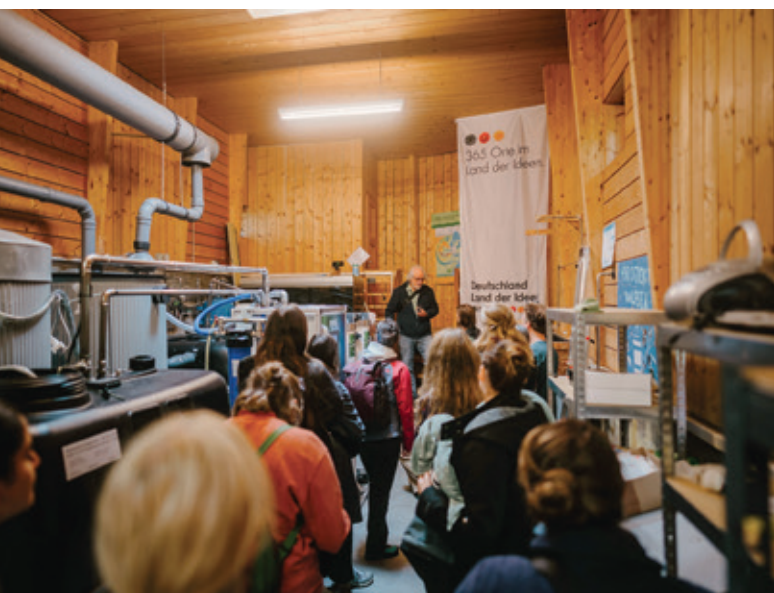
Guided tour of Roof Water Farm: Engineer Erwin Nolde explaining graywater treatment by means of filters.
